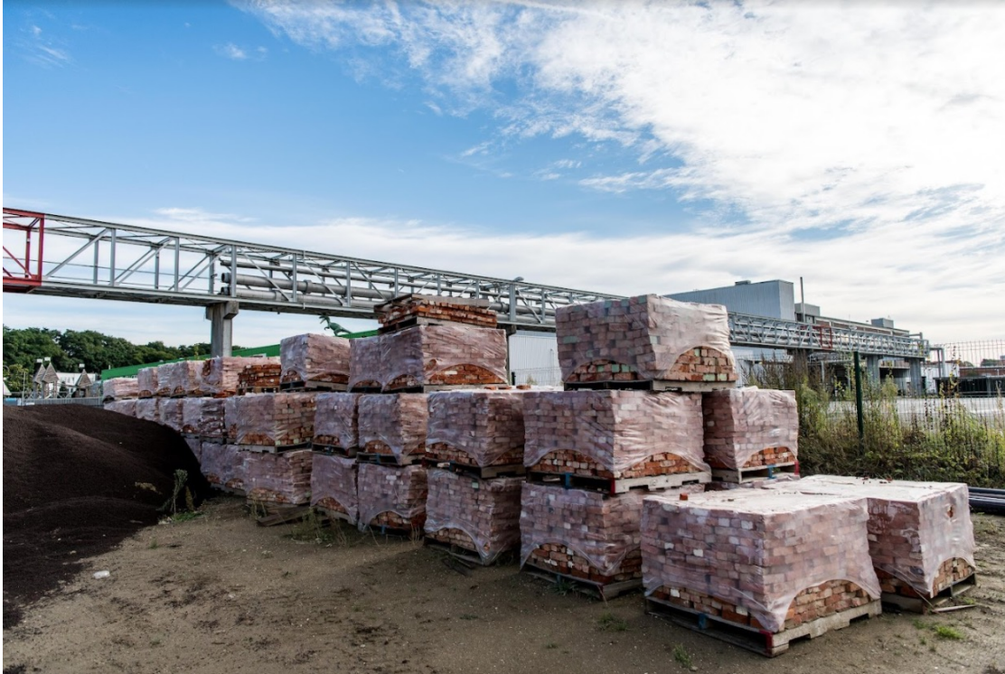
Re-use on site of cleaned brick from old warehouses
